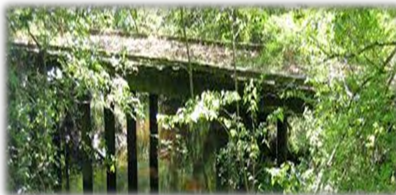
Figure 1. Old Bridge over Half Moon Creek
