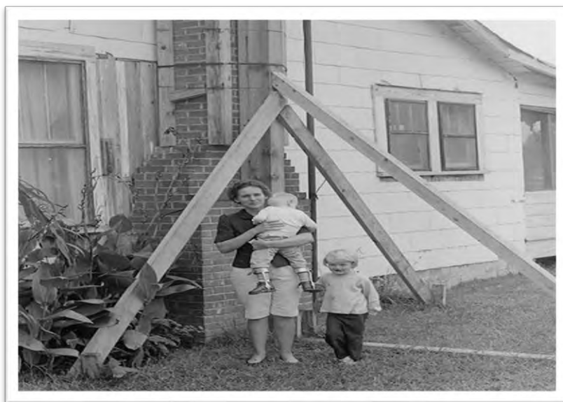
Figure 14. Residents stabilize chimneys, porches, and outbuildings in anticipation of the blast.
