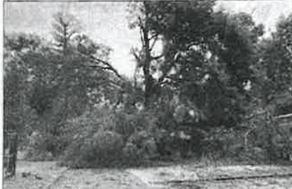
Multiple power poles were snapped in the alley between Bowles and Pecan streets, along with several large trees.
