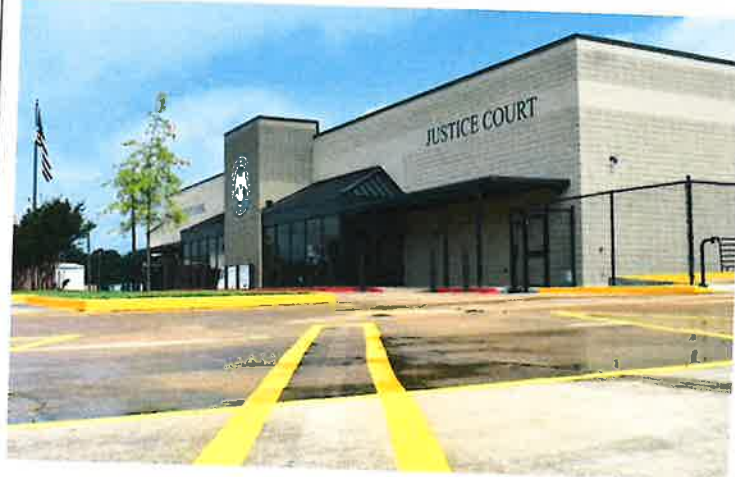
Some wiring for the security system, screens for the secure parking areas, and furniture for the inside are the only things that remain for the new Clay County Justice Center to be finished in the old Jinxey Jungle/Pass It On building on Main Street in West Point. The parking lots were striped last week and the furniture should arrive in about a month. The county may hold an open house on the $3.3 million, 20,500-square-foot facility next month before offices start moving in in August. That process may take as much as a month.
