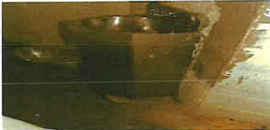
A-Zone Cell #18 and Cell #19 Leaking Water at the base
