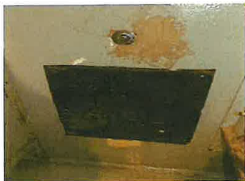
Bed 116-117 Missing Light Fixture
