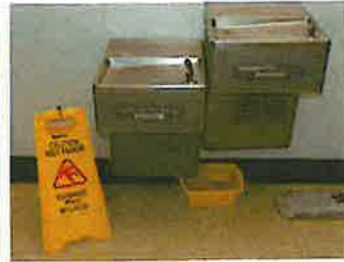
Room 229 has a water leak under the sink/ Unit 42 back desk water fountain is leaking
