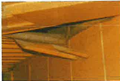
Ceiling Panel Need Replacing On B-Zone
