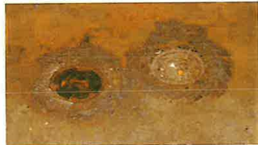
A-Zone Floor Drain was clogged
