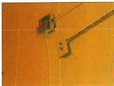
Bed 116-117 Missing Light Fixture
