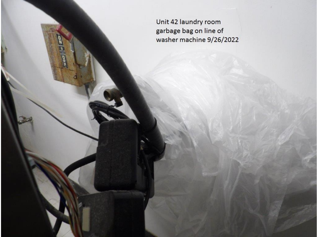
Unit #42 - Laundry Room washer line has a garbage bag tied around for leakage
