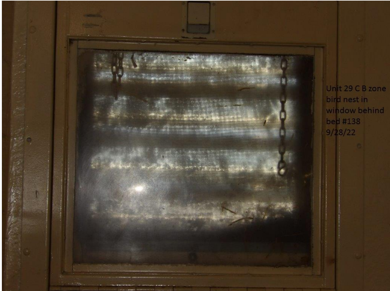
Unit #29 - C-Bldg. B-Zone cell #138 window is covered with bird nests
