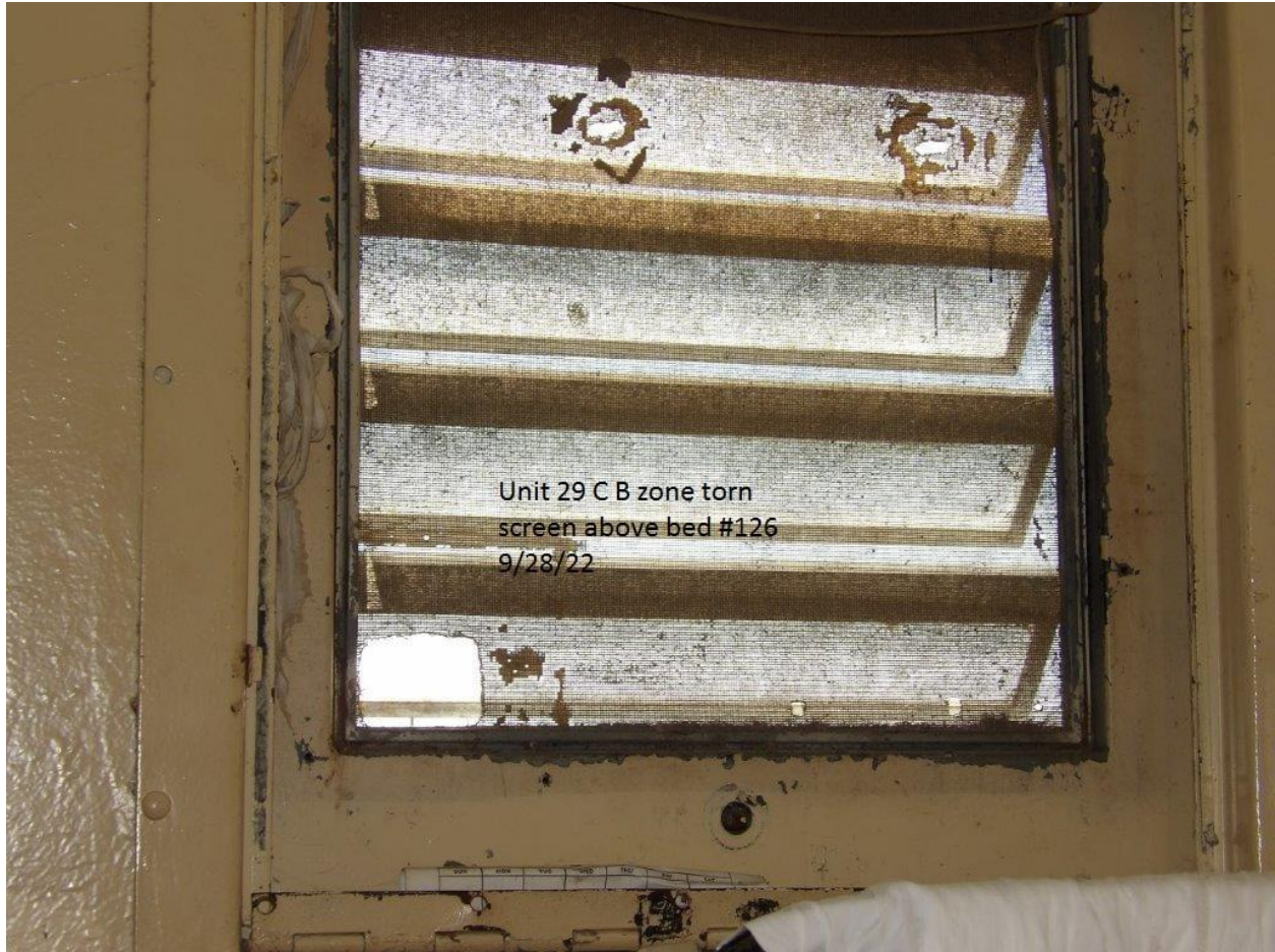
Unit #29 - C-Bldg. B-Zone cell #126 window screen is torn
