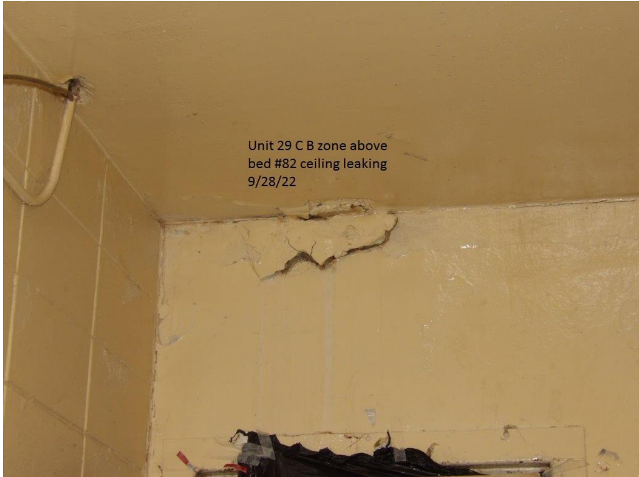
Unit #29 - C-Bldg. B-Zone ceiling leaks above Bed #82
