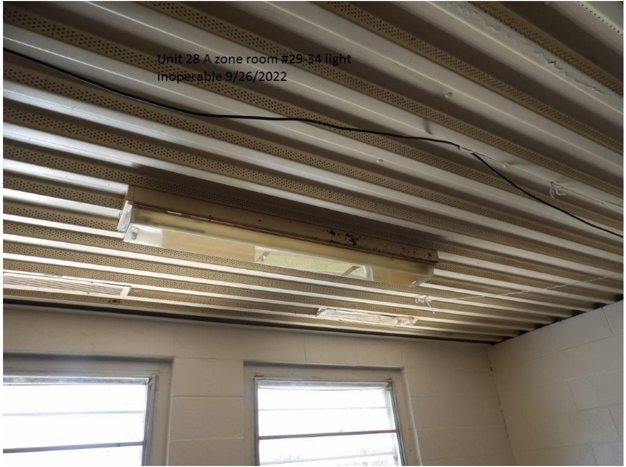
Unit #28 - A-Zone light does not work in cubicles #29-34
