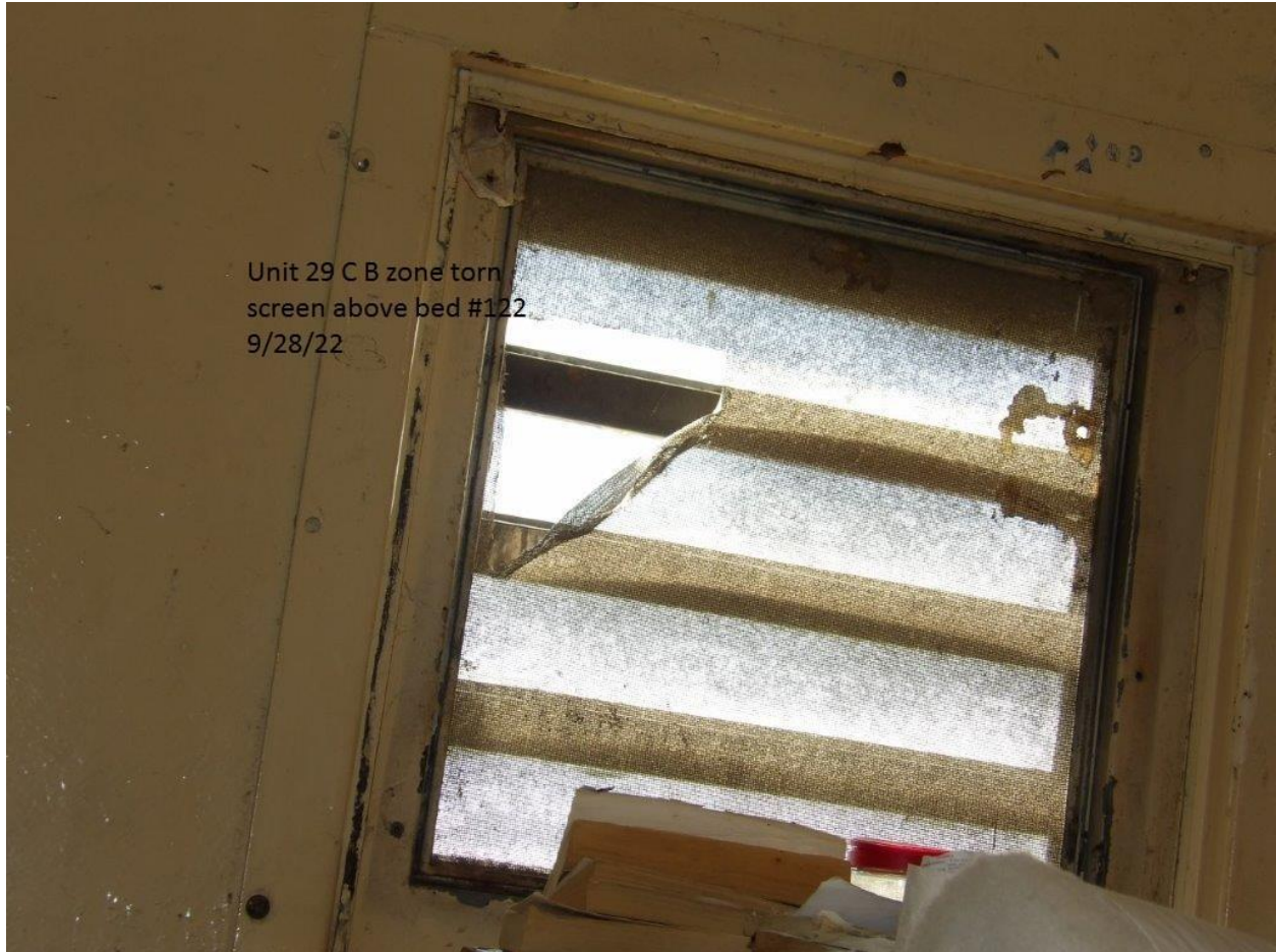
Unit #29 - C-Bldg. B-Zone cell #122 window screen is torn
