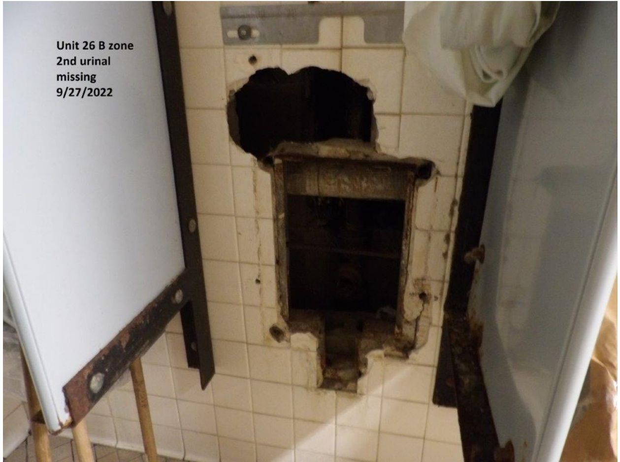
Unit #26 - B-Zone 2 nd urinal is missing and has a hole in the wall
