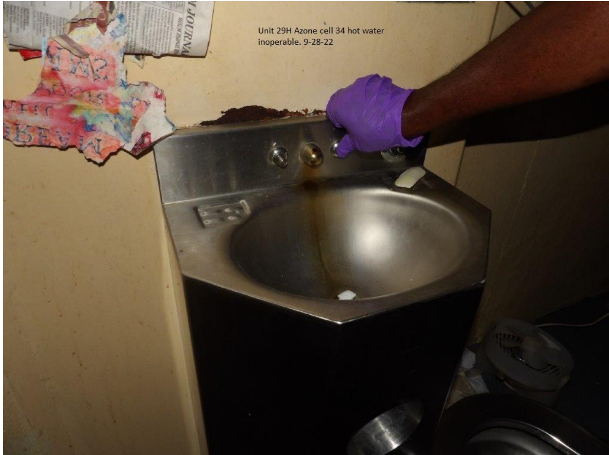
Unit #29 - H-Bldg. A-Zone cell lavatory hot water does not work
