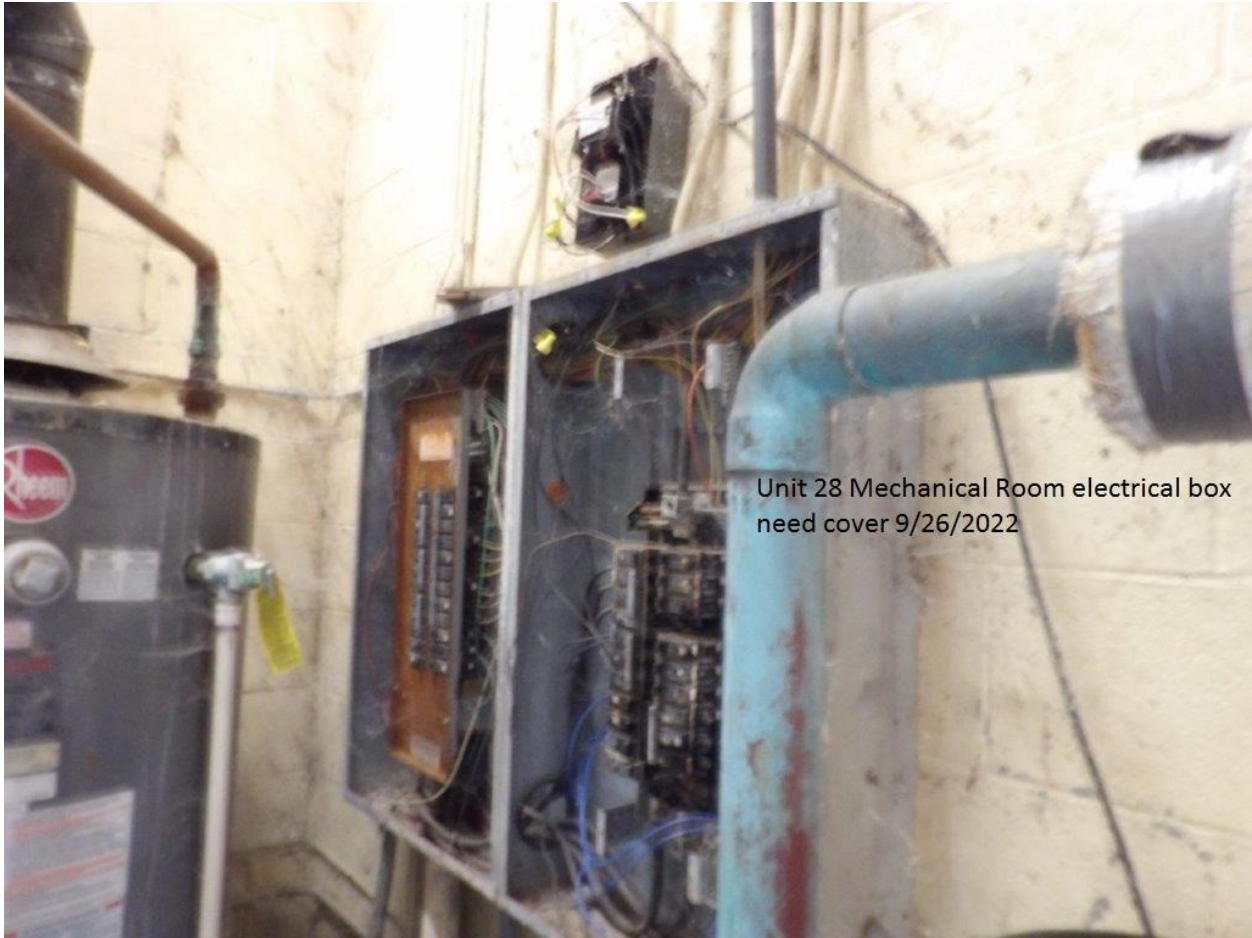
Unit #28 - Mechanical Room electrical box door cover missing
