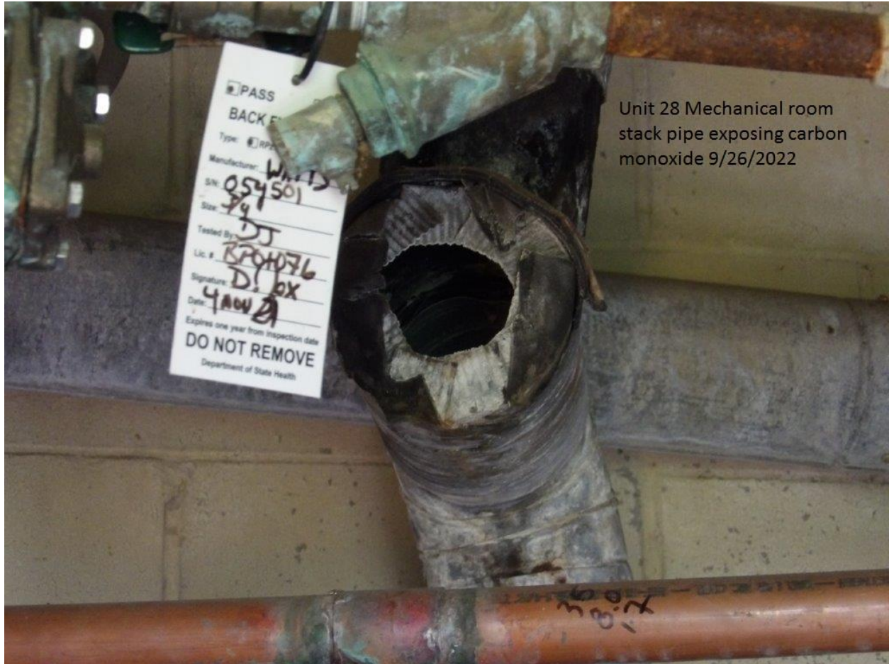
Unit #28 - Mechanical Room boiler exhaust pipe is broken and possibly exposing carbon monoxide
