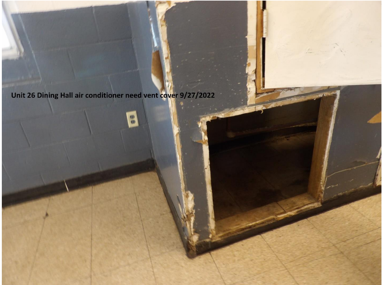
Unit #26 – The dining hall air conditioner vent cover is missing
