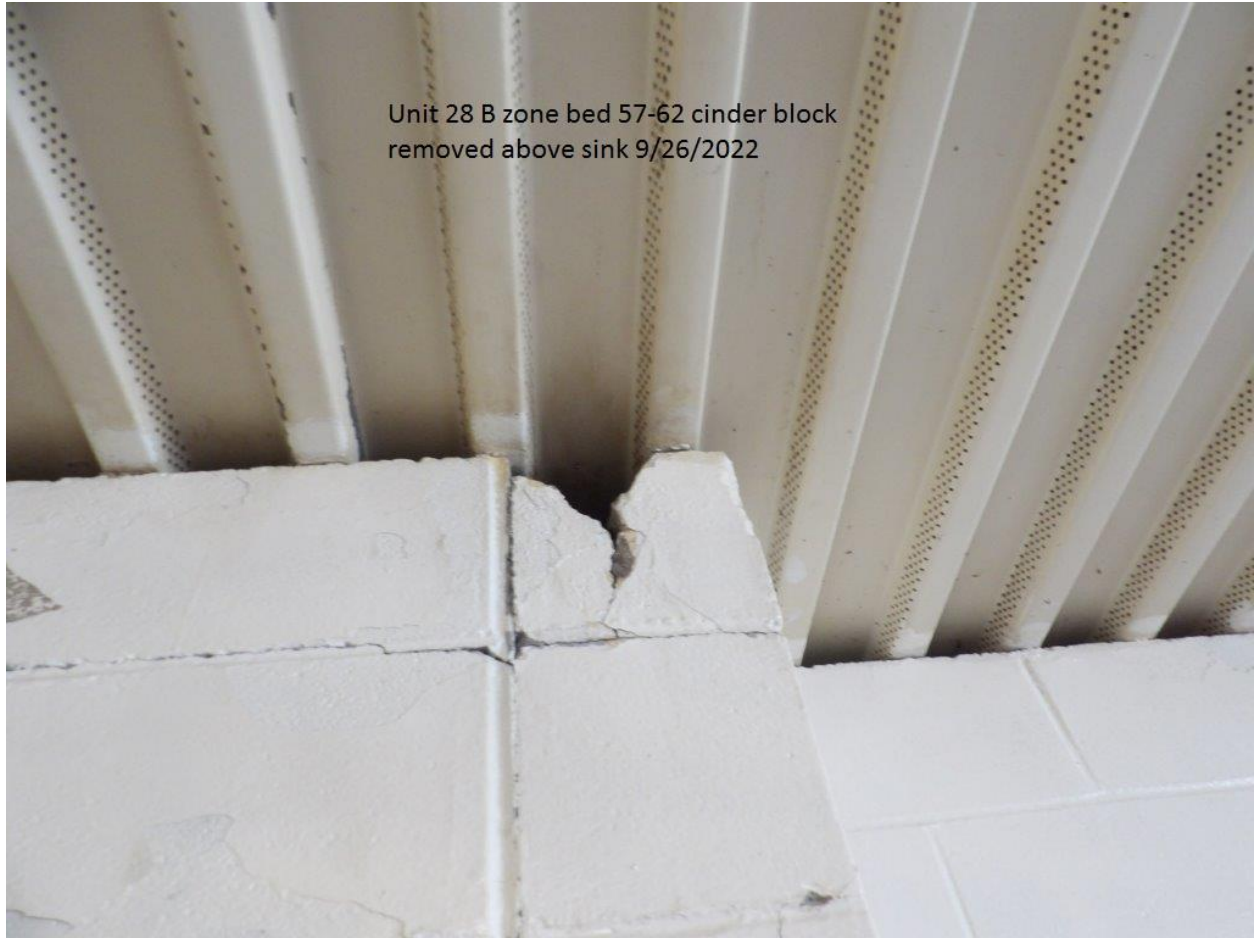
Unit #28 - B-Zone - Cinder blocks are loose from the ceiling above beds #57-62
