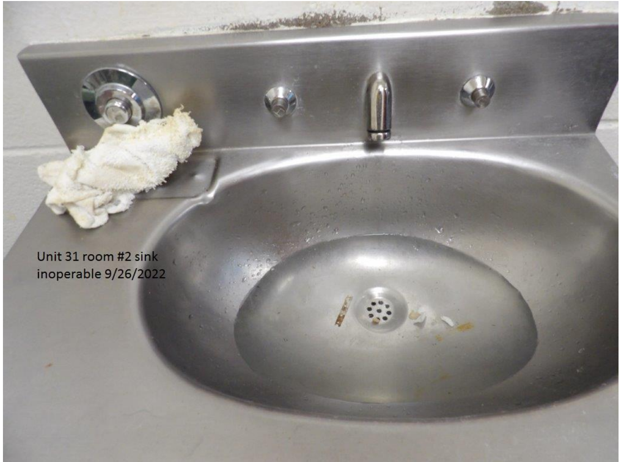
Housing Unit #31 lavatory sink is stopped up
