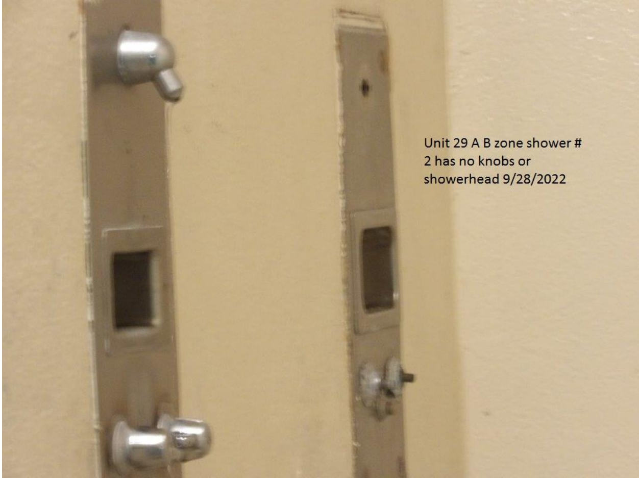
Unit #29 - A-Bldg. B-Zone 2 nd shower is missing knobs and shower head
