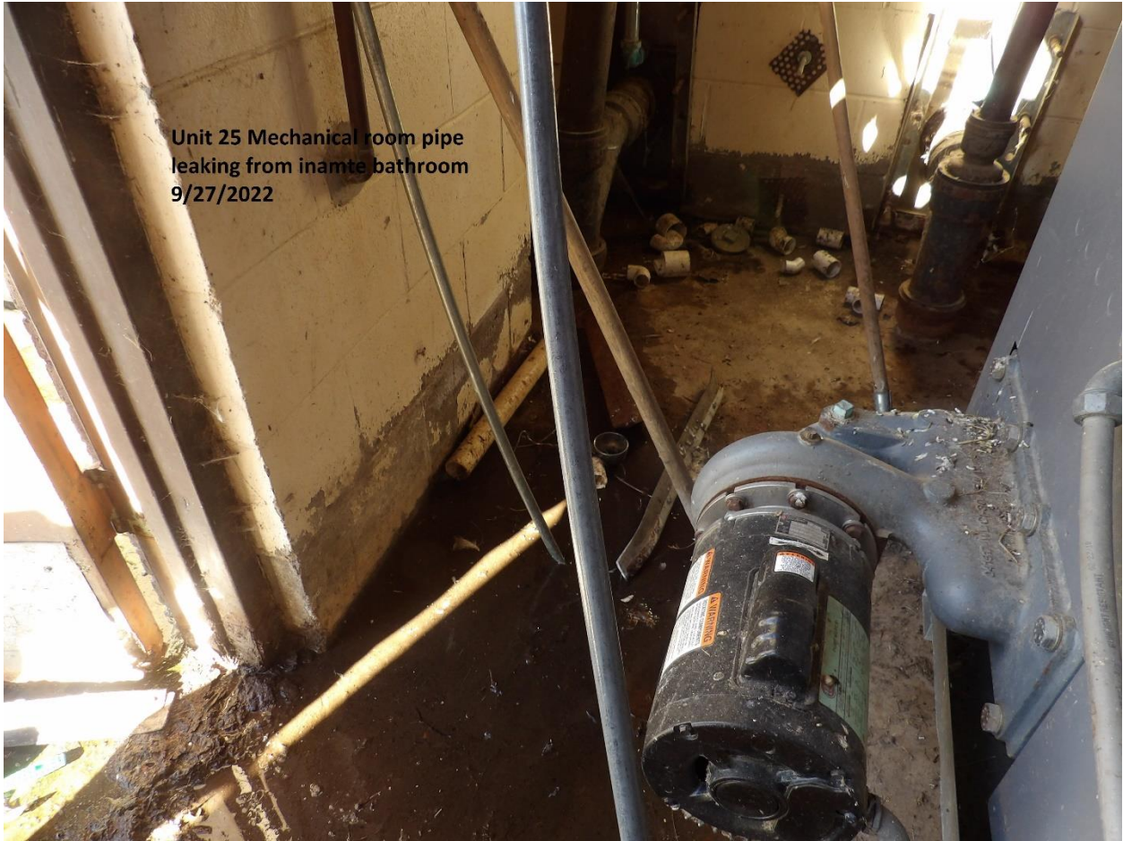
Unit #25 - Mechanical room has water leaking in from the A-Zone toilet
