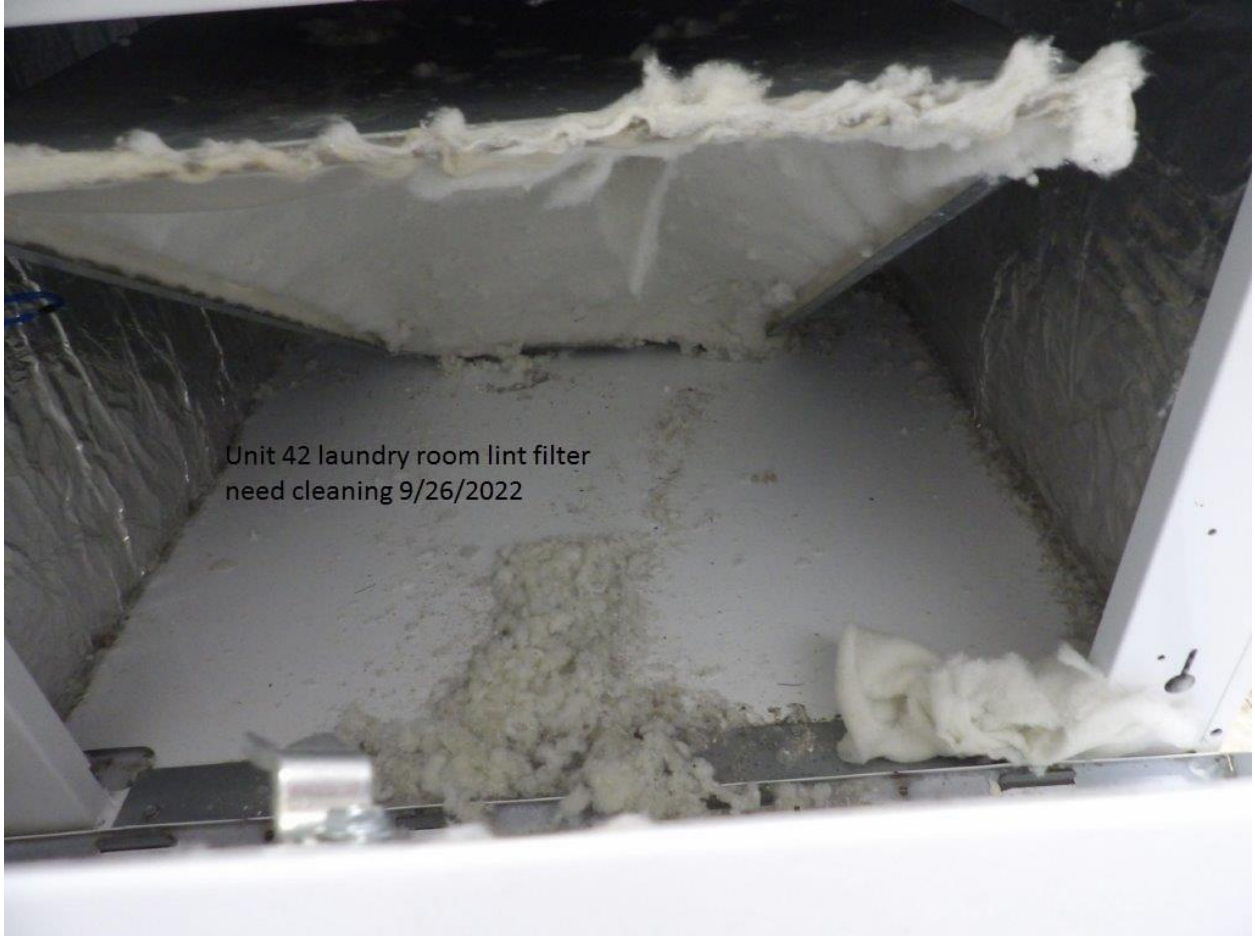
Unit #42 - Laundry Room dryer lint compartment needs cleaning
