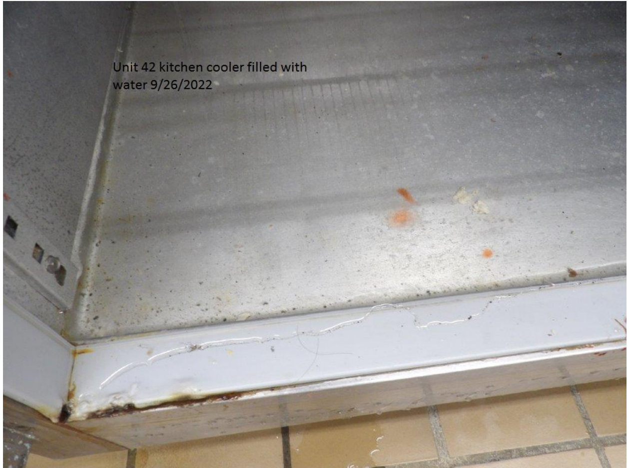
Unit #42 - Kitchen cooler is leaking water in the bottom
