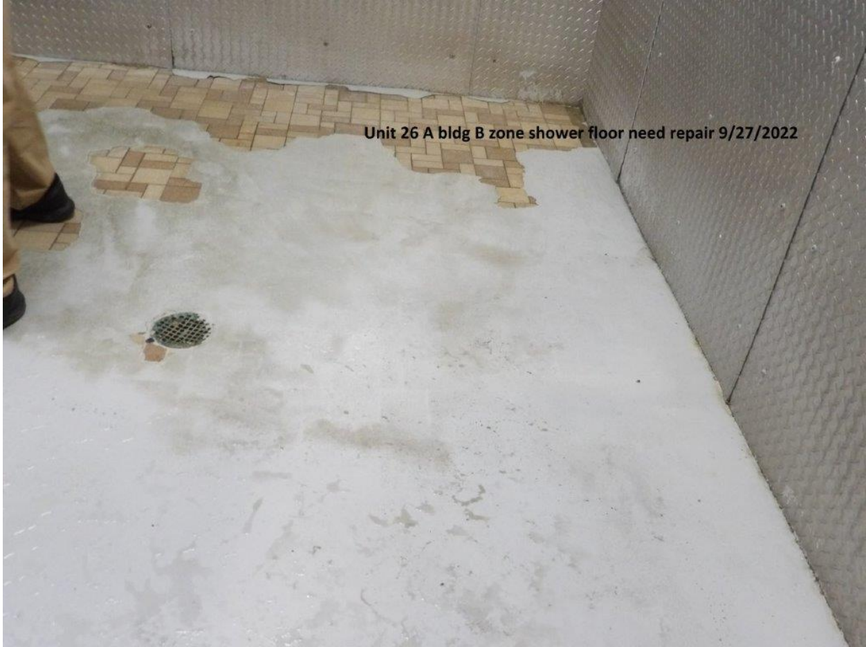
Unit #26 - A-Bldg B-Zone shower is missing tiles and holding water
