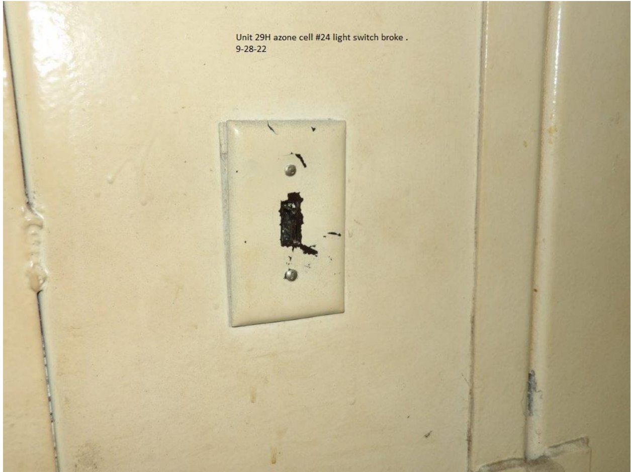
Unit #29 - H-Bldg. A-Zone cell light switch is broken
