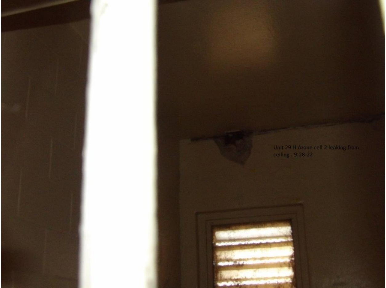
Unit #29 - H-Bldg. A-zone ceiling has a leak
