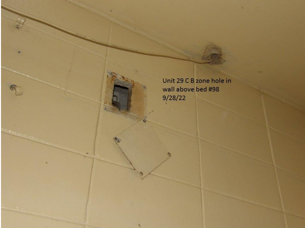
Unit #29 - C-Bldg. B-Zone wall has a hole at the top
