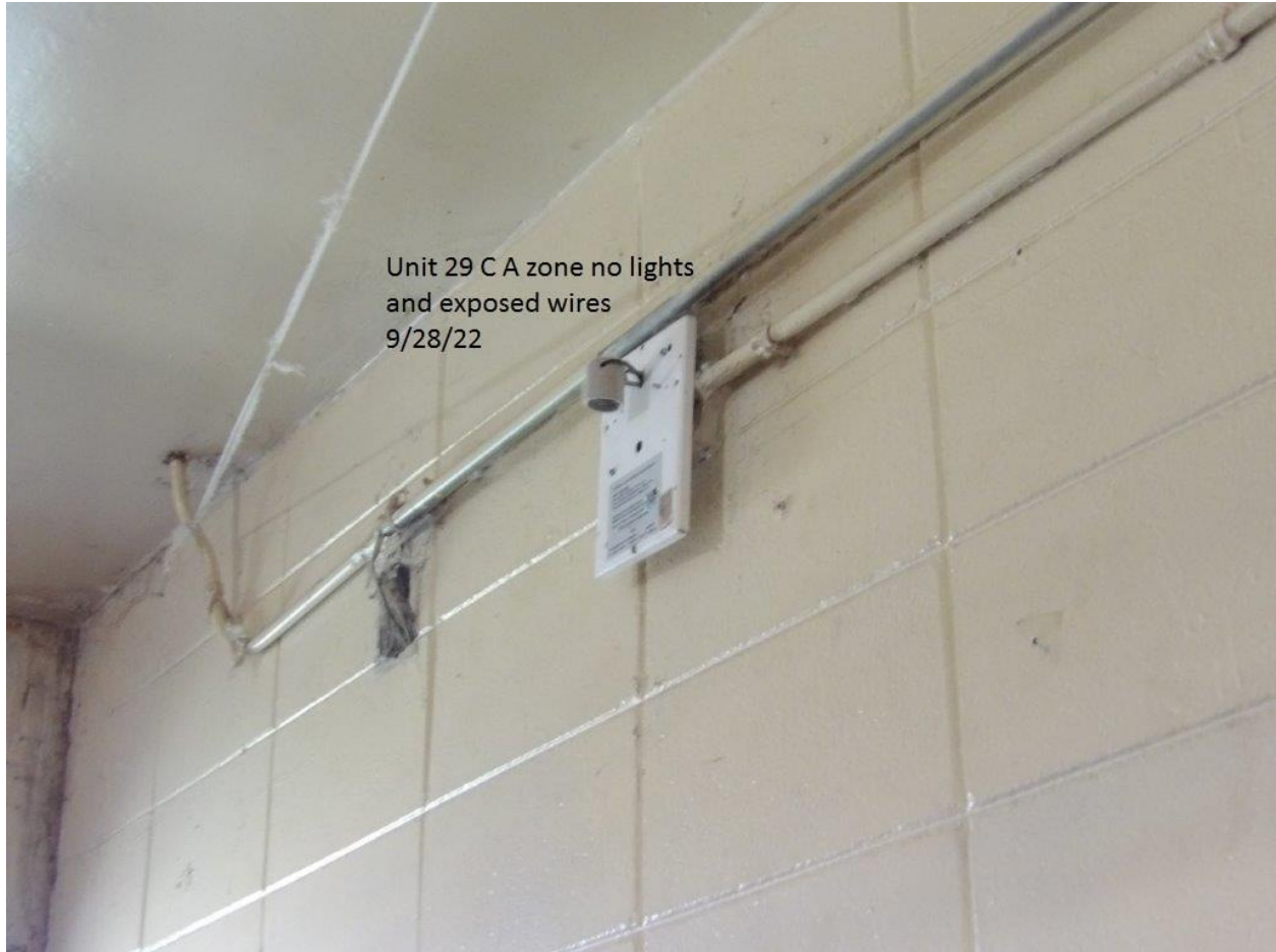
Unit #29 - C-Bldg. A-Zone light fixtures are torn out and has exposed electrical wires
