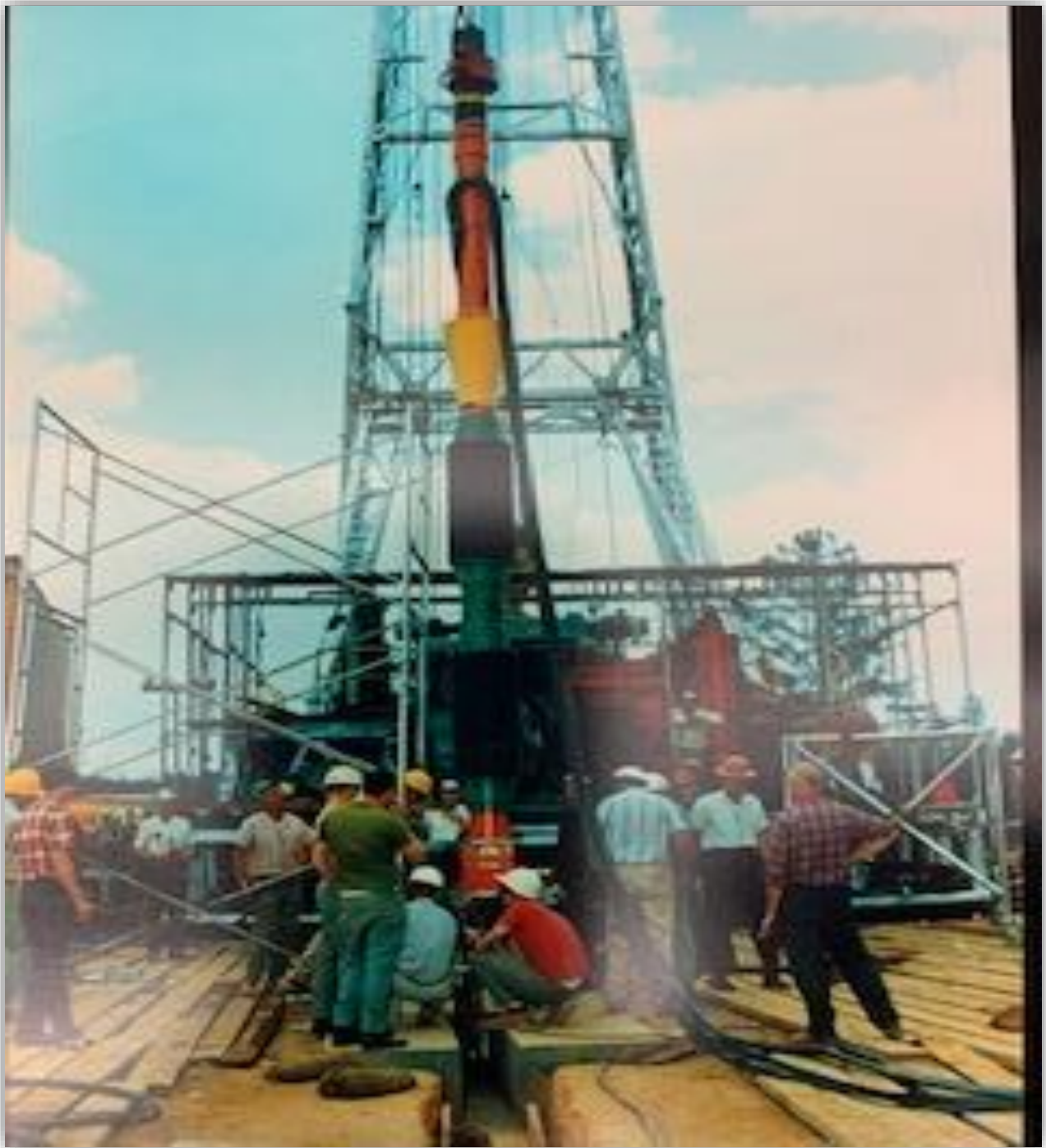
Figure 8, Sterling package going down hole
