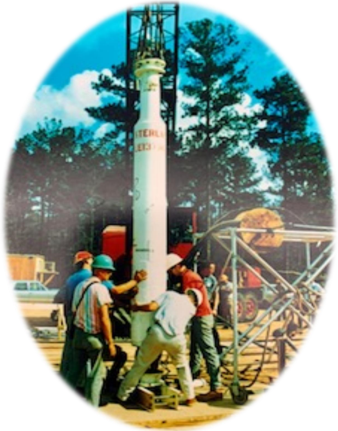
Figure 4, Sterling package going down hole
